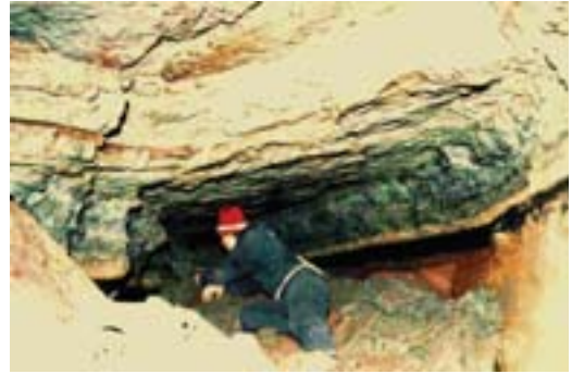
Fig. 3. Sablino Complex Monument. Levoberezhnaya Mine, the collapsed hall
