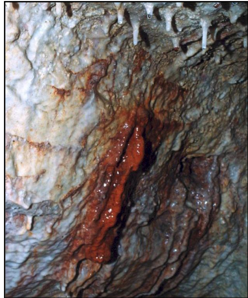
Fig. 17. Calcite dripstones in the sandstone of the Szénlopó Tunnel, Hungary (photo by L. Buda)
